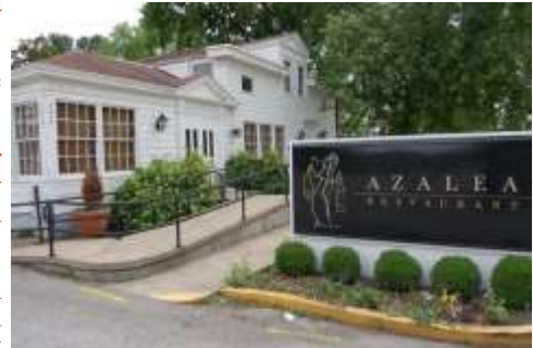
The building that housed the old Bauer's and Azalea restaurant currently is slated for demolition.
